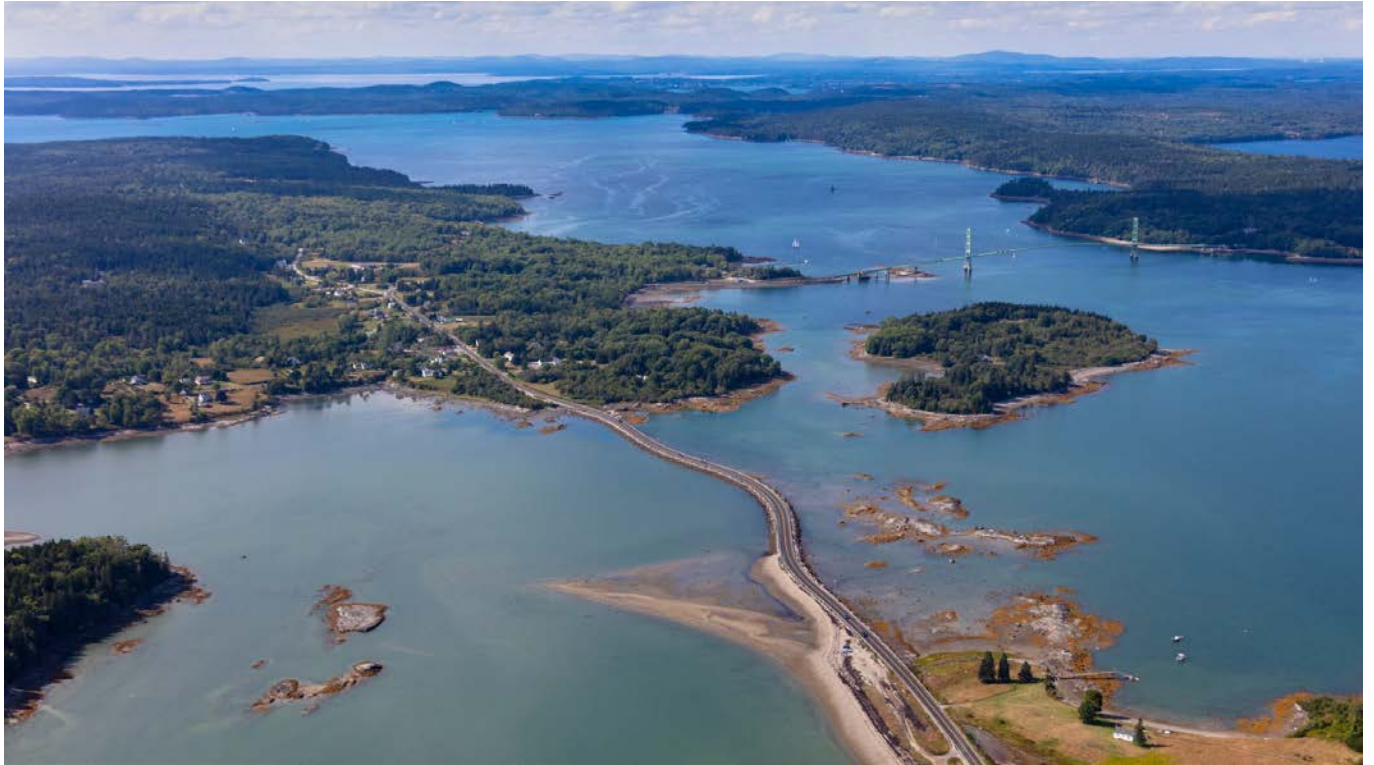
The Deer Isle Bridge (top right) connects the archipelago to the mainland. The main link between Little Deer Isle and Deer Isle is a half-mile-long causeway that already sees frequent flooding during storms. Photo by Alex MacLean.
